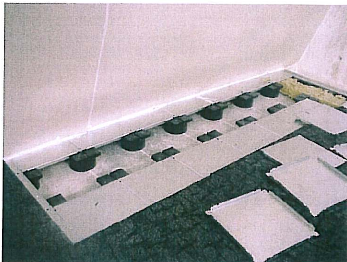
figure 5a: floor under construction
